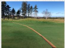
Sod cutting trenches and installing black drain pipe to attract sunlight and use the trenches to move water off the green during melts
